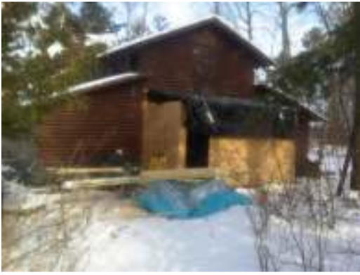
Wrens cabin with a new bathroom extension under construction
