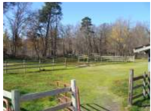
Lots of corral fence repaired and replaced
