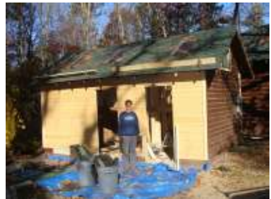
Junior bathroom near Happy Hollow, is being remodeled
