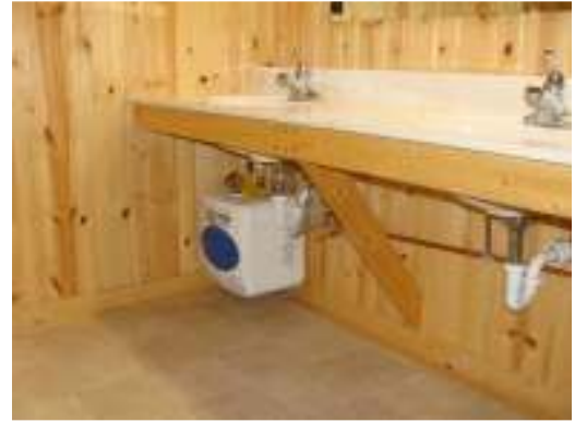
Hot water heaters added to an additional 8 cabins at camp
